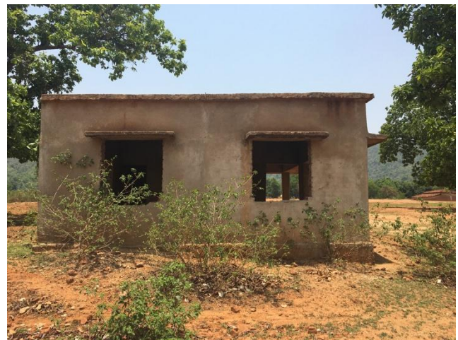
Under construction hollang Anganwadi from 2007
